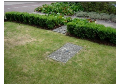
PHOTOGRAPH 3 EXISTING BT AND VODAFONE CHAMBERS IN PLANTED AREAS OUTSIDE 3 / 4 LINDENWOOD
