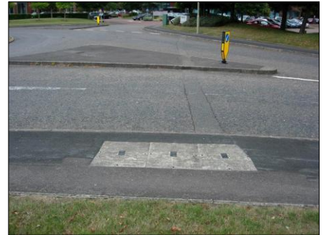
PHOTOGRAPH 6 EXISTING VODAFONE CHAMBER AT JUNCTION OF CROCKFORD LANE WITH LIME TREE WAY
