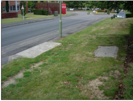
PHOTOGRAPH 1 BT CHAMBERS IN VERGE AND FOOTWAY ON CROCKFORD LANE (EAST SIDE) OUTSIDE MAPLEWOOD
