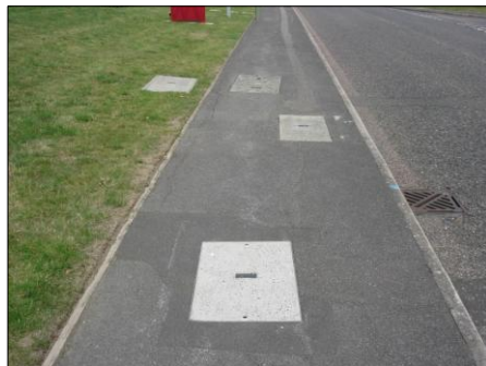
PHOTOGRAPH 11 EXISTING BT, VIRGIN MEDIA AND VODAFONE CHAMBERS ON LIME TREE WAY OPPOSITE JUNCTION WITH STAG OAK CLOSE
