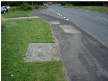
PHOTOGRAPH 1 EXISTING BT AND VODAFONE CHAMBERS ADJACENT LINDENWOOD IN CROCKFORD LANE
