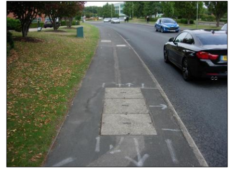
PHOTOGRAPH 3 BT, VIRGIN MEDIA AND VODAFONE CHAMBERS IN FOOTWAY ON CROCKFORD LANE (WEST SIDE) OUTSIDE PINEWOOD
