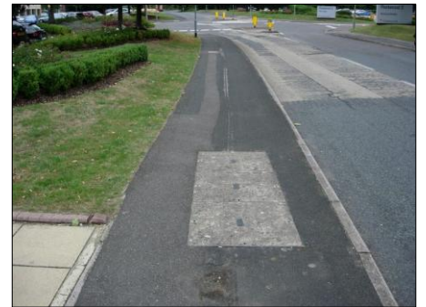
PHOTOGRAPH 9 EXISTING BT AND VIRGIN MEDIA CHAMBERS ON CROCKFORD LANE AT JUNCTION WITH REDWOOD ACCESS ROAD
