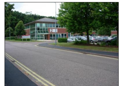
LOOKING WEST ALONG ACCESS TO ESTATE
