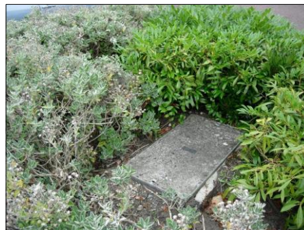
PHOTOGRAPH 2 EXISTING BT AND VODAFONE CHAMBERS IN PLANTED AREA ADJACENT TO 1 LINDENWOOD
