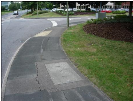
PHOTOGRAPH 7 EXISTING VODAFONE CHAMBERS ON CROCKFORD LANE AT JUNCTION WITH REDWOOD ACCESS ROAD
