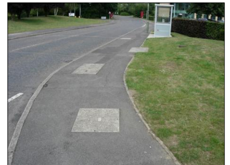
PHOTOGRAPH 12 EXISTING BT AND VIRGIN MEDIA CHAMBERS ON LIME TREE WAY ADJACENT JUNCTION WITH STAG OAK CLOSE
