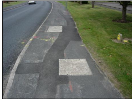
PHOTOGRAPH 2 VIRGIN MEDIA AND VODAFONE CHAMBERS IN FOOTWAY ON CROCKFORD LANE (EASTSIDE) OUTSIDE MAPLEWOOD
