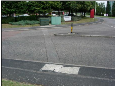
PHOTOGRAPH 4 EXISTING BT AND VIRGIN MEDIA CHAMBERS AND CABINETS AT JUNCTION OF CROCKFORD LANE WITH LIME TREE WAY
