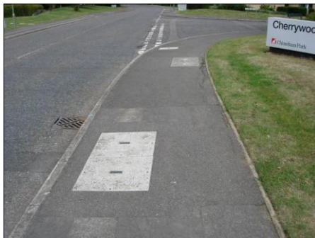
PHOTOGRAPH 10 EXISTING VIRGIN MEDIA CHAMBERS IN FOOTWAY ON LIME TREE WAY AT JUNCTION WITH STAG OAK CLOSE
