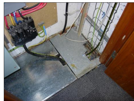
PHOTOGRAPH 6 EXISTING BT INTAKE LOCATION BENEATH FLOOR IN RISER CUPBOARD, ASSUMED ONE DUCT
