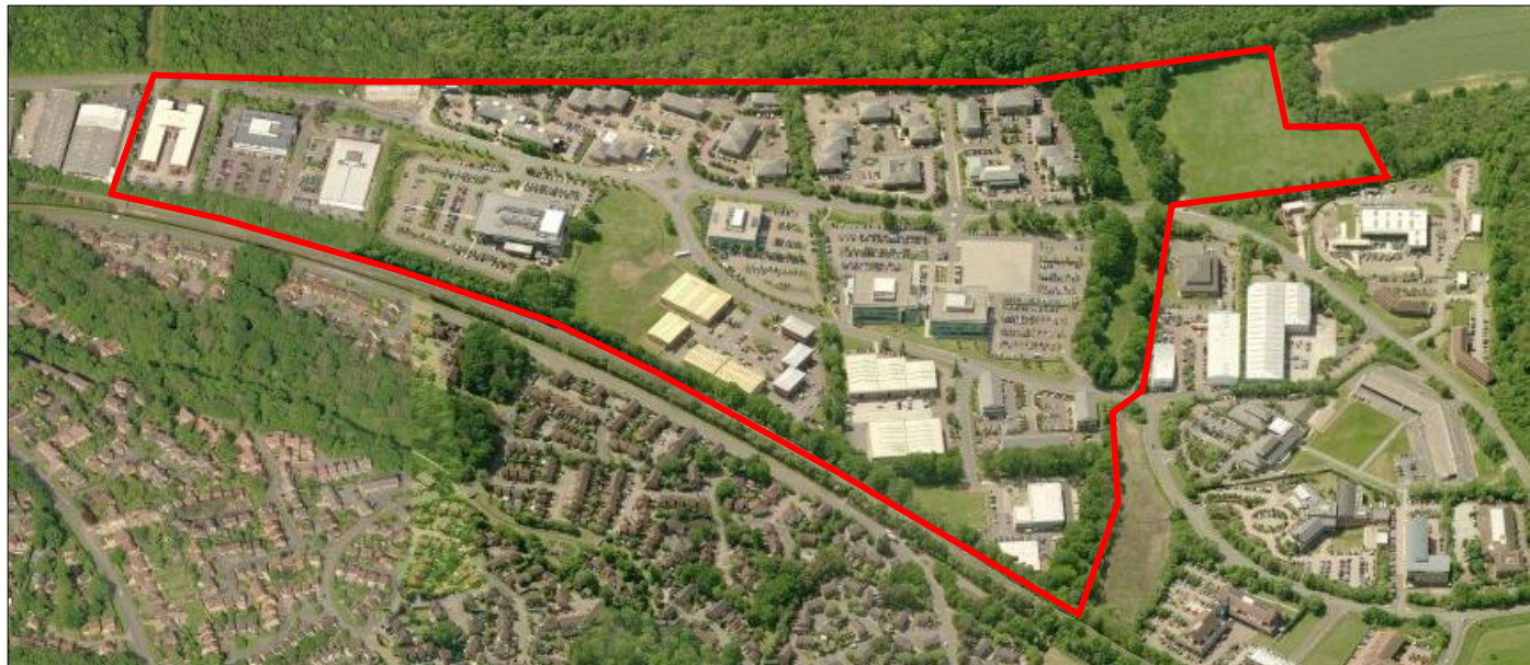
SITE AERIAL VIEW (Site extent highlighted in red)
