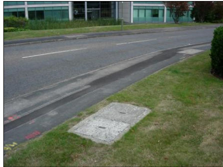
PHOTOGRAPH 5 EXISTING EASYNET AND VODAFONE CHAMBERS AT JUNCTION OF CROCKFORD LANE WITH LIME TREE WAY
