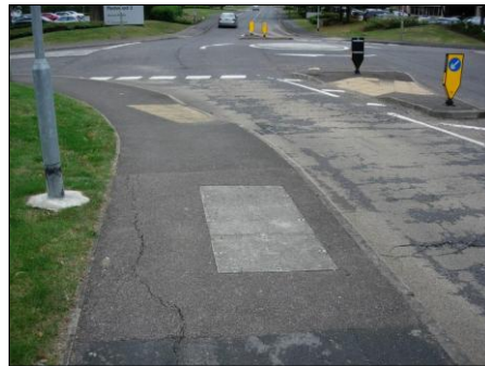
PHOTOGRAPH 8 EXISTING VODAFONE CHAMBER ON CROCKFORD LANE AT JUNCTION WITH REDWOOD ACCESS ROAD
